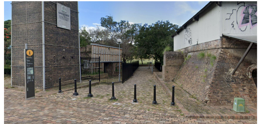
Main pedestrian entrance to kilns
